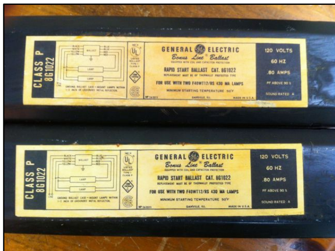
Suspected PCBs Ballasts
